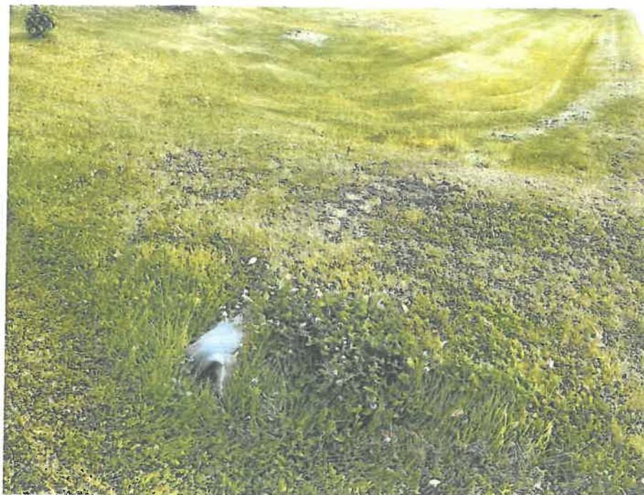
C102 – DAMAGED END
