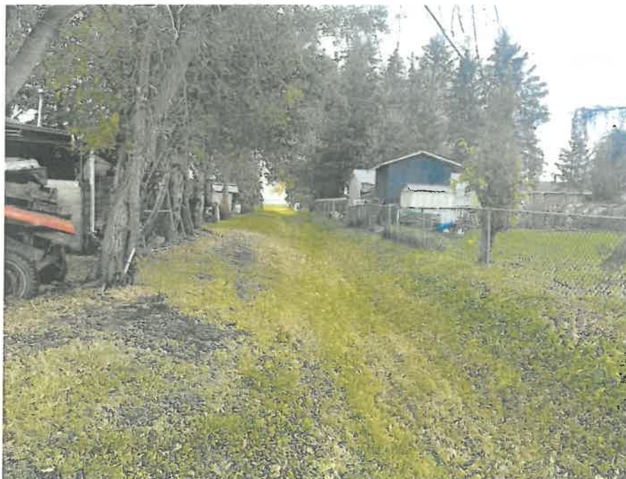
DRAINAGE CHANNEL RUNNING NORTH BETWEEN LAKEVIEW DRIVE LOOP
