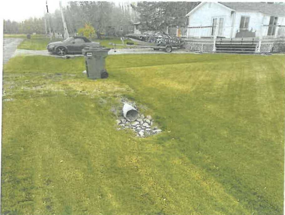
C210 – TYPICAL RESIDENTIAL APPROACH ALONG LAKEVIEW DRIVE
