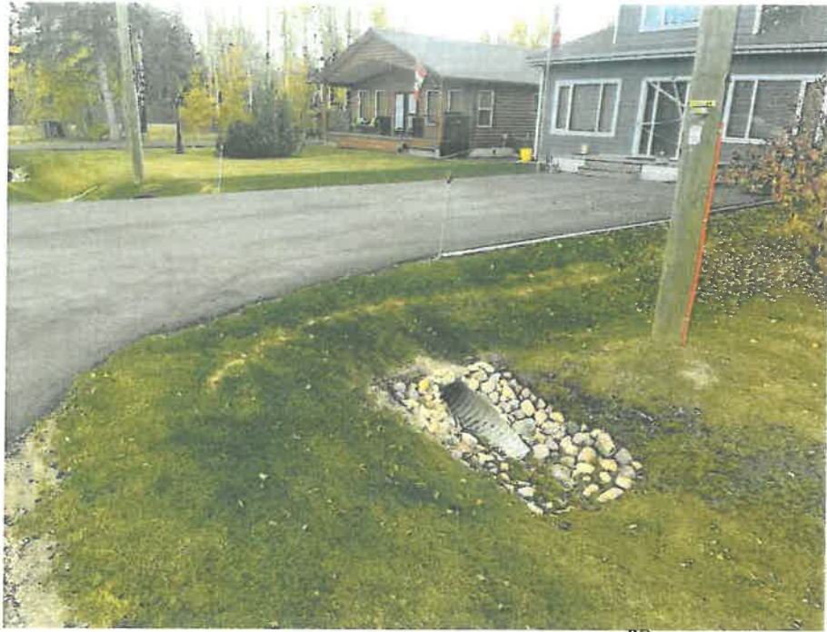
DITCHES AND APPROACHES ALONG 63 RD STREET
