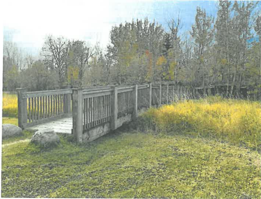
BRIDGE OVER CHANNEL FOR LOT LP
