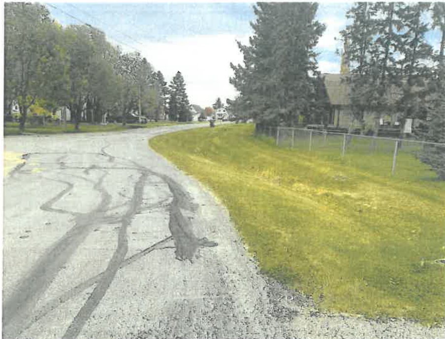
DITCH SYSTEM ALONG 64 TH STREET
